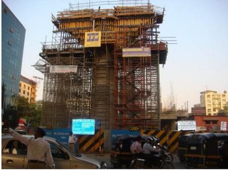
the high rate of reinforcement, introduction of few transverse prestressing cables. To complicate more this state, the installation of fixed pot bearings with dispositions to create a fixed point for seismic event, or for braking and acceleration loads at the top of pier cap, obliged the contractor to work slowly with a great awareness in all stages of pouring, and
