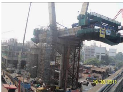
*Fig. 25 : Scaffolding for the anti-uplift pier*
