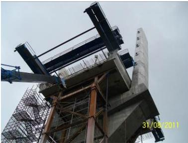
After the realisation of the pier cap and the pouring of the pylons with its incorporated saddles, the works of the deck began with the installation of the lateral scaffolding and temporary tie down as we see in fig. 21: the form traveler is in progress, and the bents with the temporary tie down including an active stay cable to assure the
