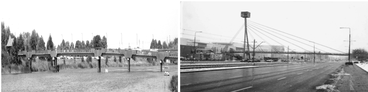
Fig. 7. Bridge over Nogat river in Malbork and over Woloska street in Warsaw.
