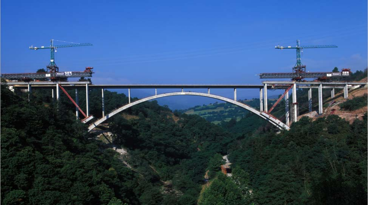
Figure 17. View of Cieza viaduct
