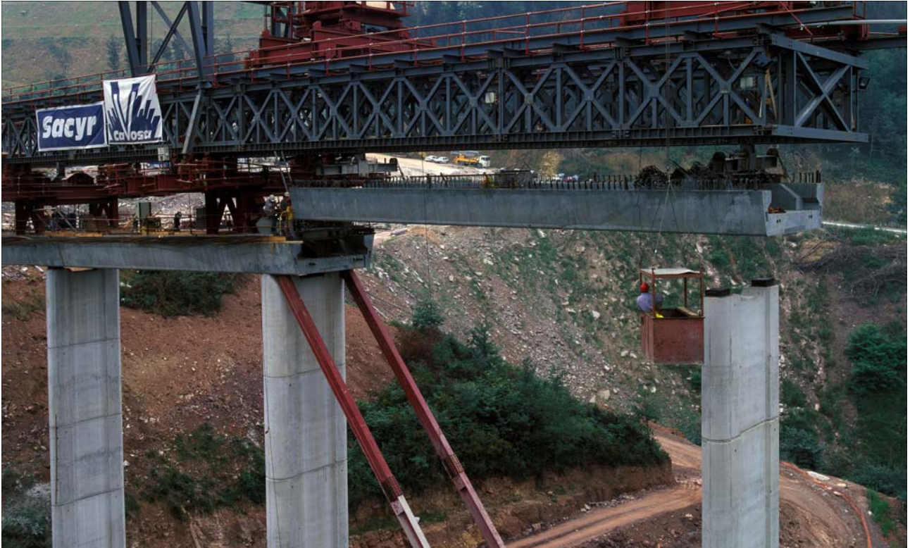
Figure 7. Launching of precast beam
