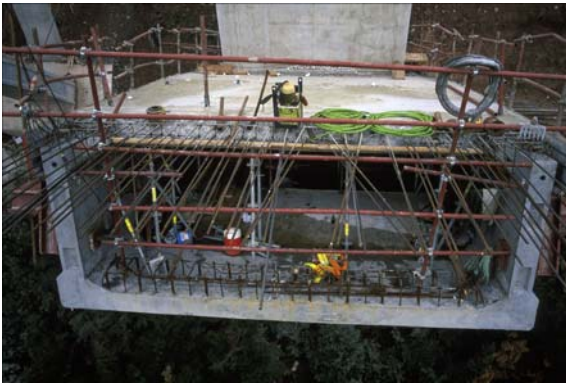
Figure 2. Front view of arch segment
