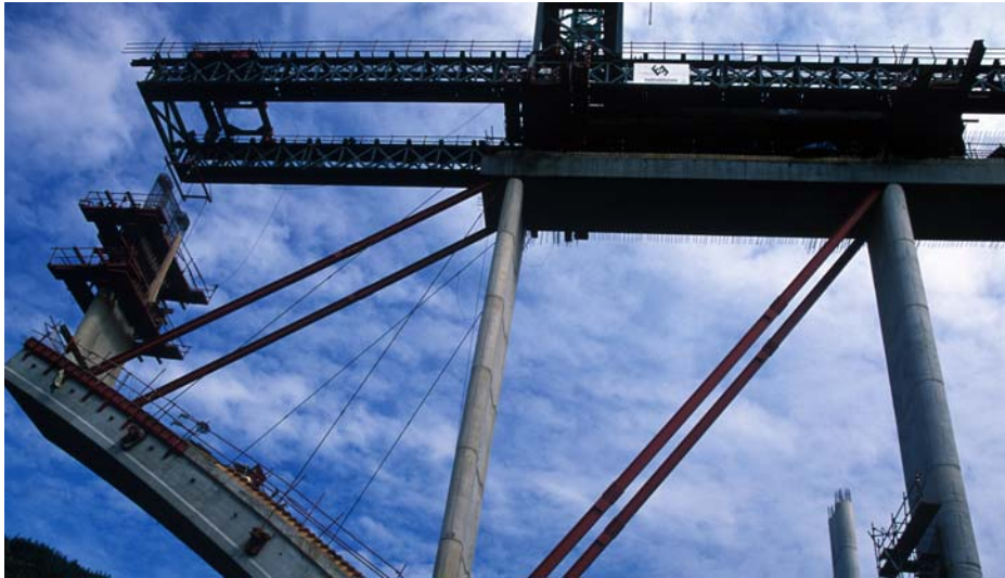
Figure 1. View of semi-arch during construction
